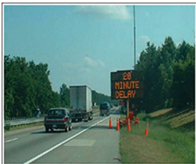
Figure 3.19 Roadside message sign providing delay information (Bushman & Berthelot, 2005).
